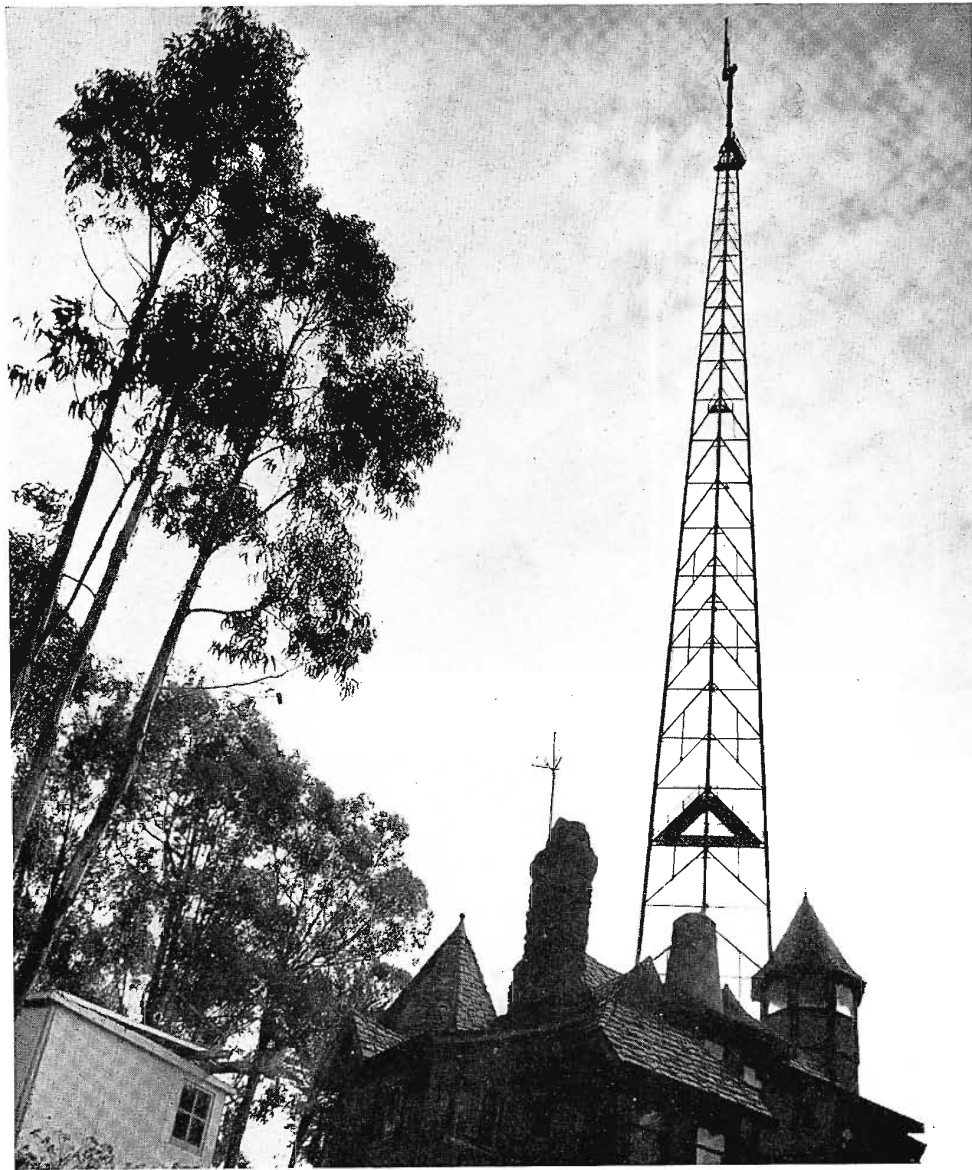
FIG. 1 (at left). The 450-foot TV-FM antenna and tower is the only outward sign of the transition of the fabulous Sutro Mansion into the ultra-modern home of KGO-TV.
