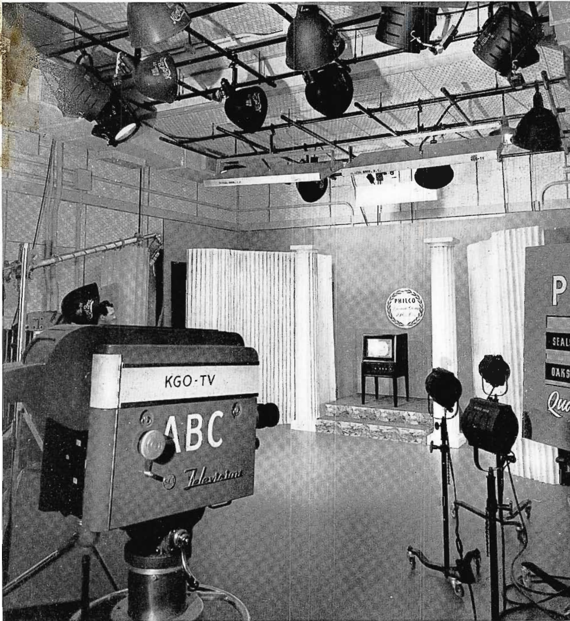
FIG. 5. View of KGO-TV's studio A. Walls and ceilings are covered with fiberglass bolts between steel studs, covered with glass cloth and chicken wire. The floor is linoleum over inch boards.
