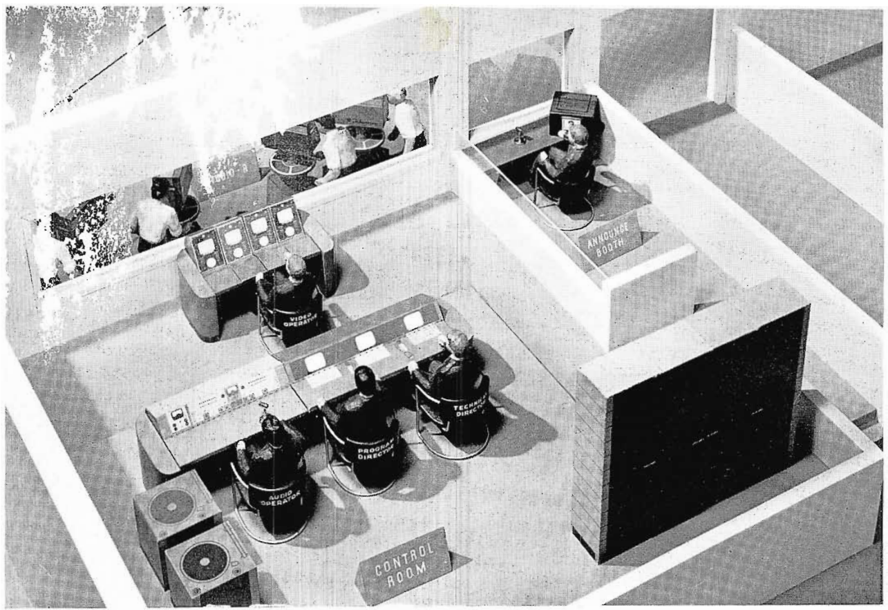
FIG. 5. Studio Control Room facilities of Fig 4, arranged with the Audio and Video Consoles on a raised platform.
